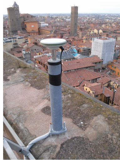
Figure 2. The BOGA GNSS antenna installed on the top of Garisenda tower by the DICAM department since 2013.
