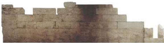
Figure 5: Three meters high corridor. The dark part was under shadow and processed with wallis filtering, prior to mosaiking
