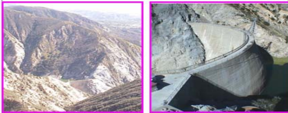
Figure 4 : Pacoima dam view
