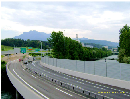
Fig. 7a): Highway bridge near Lucerne after enlarging during construction phase.
