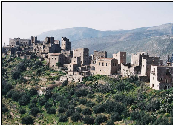
fig.1: The traditional settlement of Vathia, Stone buildings in Mani, Greece (photo by Venia Apostolidi)
