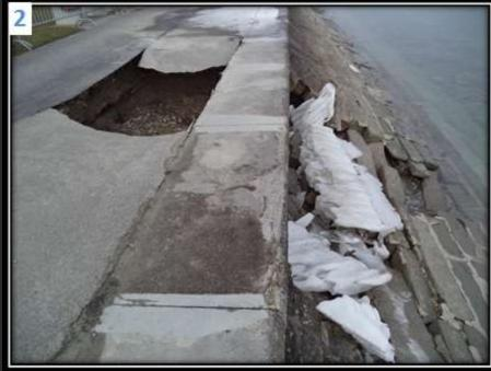
Ice shield on the shore in February (left) and collapsed ground after melting of the ice in March 2018 (right)
