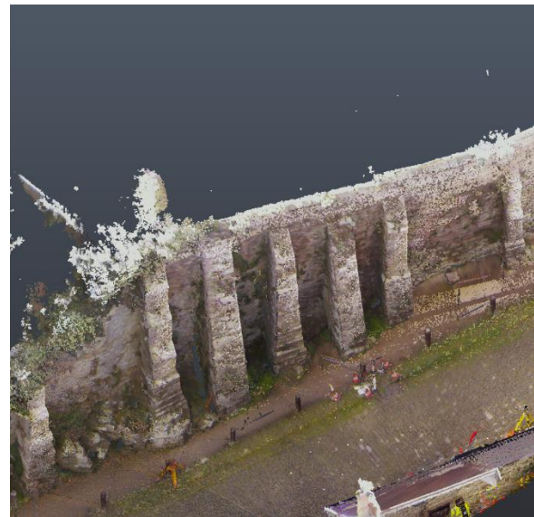
Figures 11 & 12. Final 3-dimensional model of the retaining wall at Gold Hill viewed in Autodesk ReCAP
