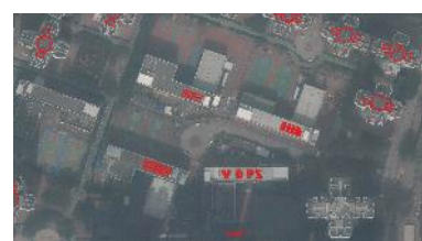
(c) Roof Tops of School
