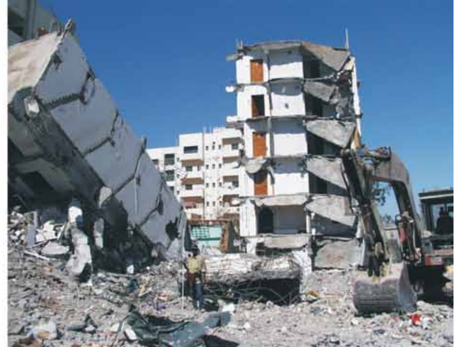
Figure 1: Examples of buildings affected by the 2001 Gujarat earthquake: (Left) heavily damaged residential building, (Right) multi-storey building that has fallen on one side (Bhuj, India) (Image courtesy by M. Markus, 2001)
