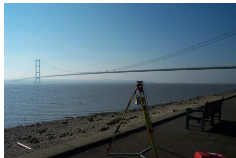
Figure 6 - The Humber Bridge showing a GPS receiver reference station in the foreground.
