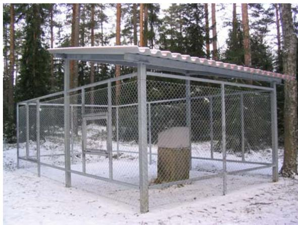
**Fig. 3.** The shelter for observation pillar and underground marker at 864 m.
