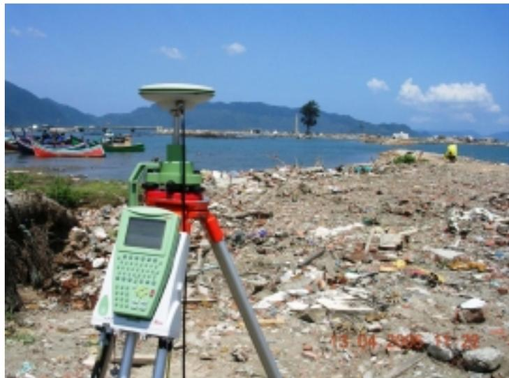
**Figure 7(a).** Example of parcel boundary reconstruction in Aceh with GPS.
