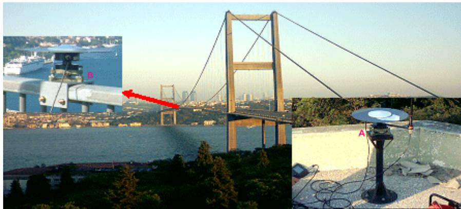
**Figure 2** Reference and object points used for measurement of Bosphorus Bridge responses under different load.
